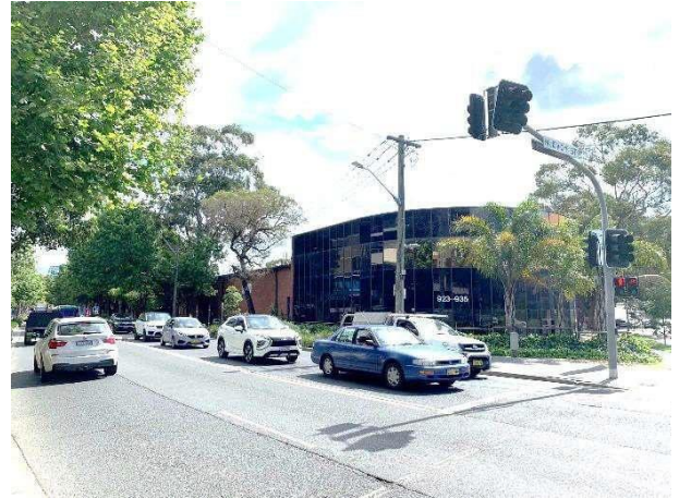
View looking south on Bourke Street along frontage of site
